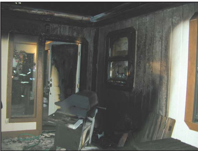
Figure 23-26 Every attempt should be made to preserve the room of origin and any significant fire patterns until after the investigators have completed their work.
