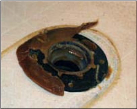
Figure 23-19 Removing a toilet and the wax ring can create a floor drain to remove large quantities of water
