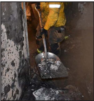
Figure 23-21 Debris carriers and scoop shovels are essential pieces of equipment used during overhaul.
